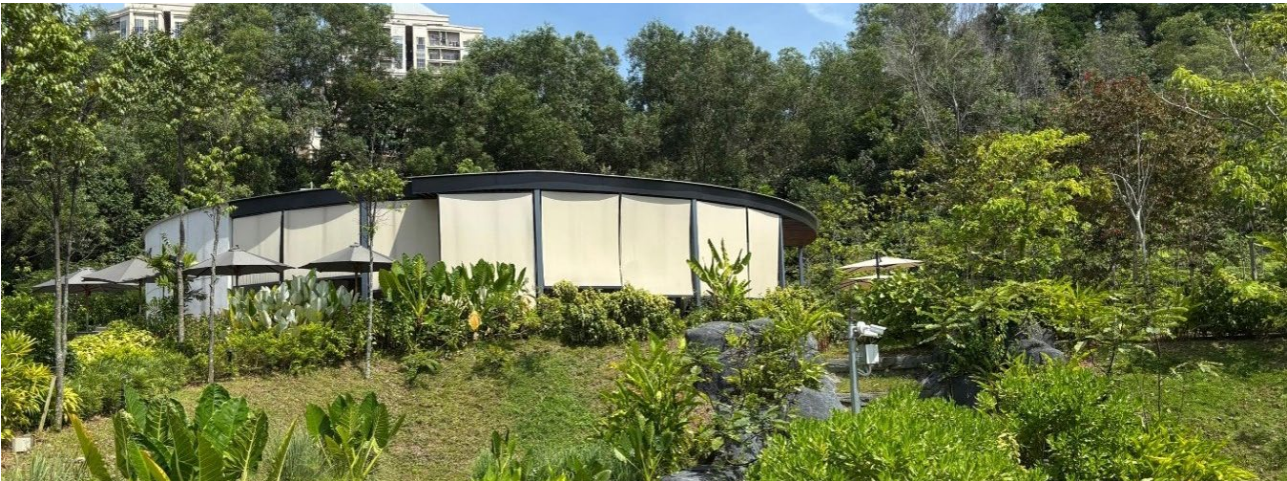
Rainwater harvesting tank
