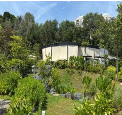
Rainwater harvesting tank
