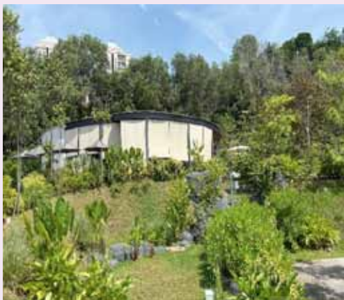
Rainwater harvesting tank
