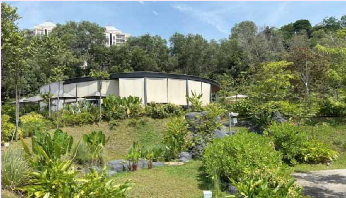
Rainwater harvesting tank
